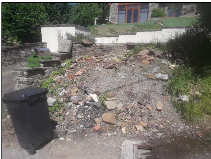
Figure 13: Evidence of debris removed from 'Culvert Inlet 1' post event (captured by Council appointed contractor during CCTV surveying operations on 30/07/2020)
