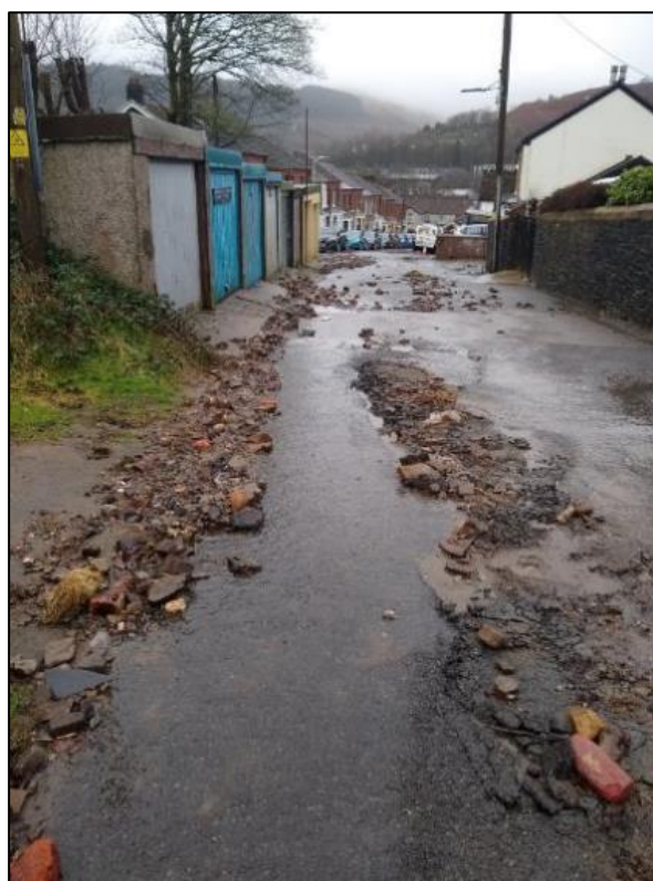
Figure 27: Road damage and debris deposited along Column Street by the surcharging ordinary watercourse flows during the storm event (image provided by resident)
