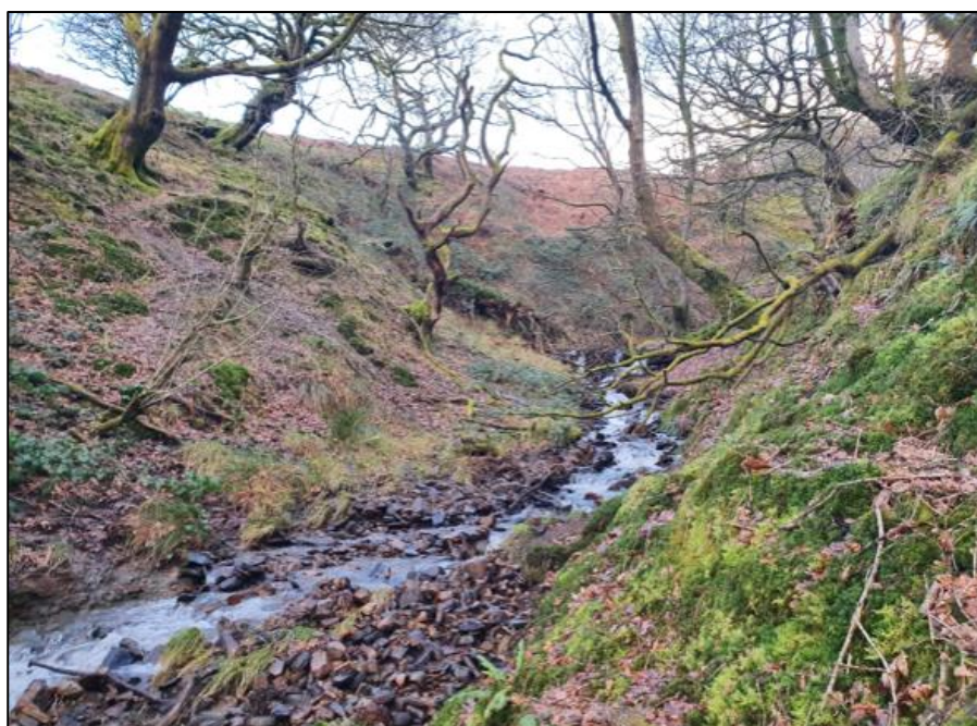
Figure 21: Photo of the unnamed ordinary watercourse upstream of 'Culvert Inlet 2' within the upper catchment (captured by RCT's Flood Risk Management team on 17 th February 2020)
