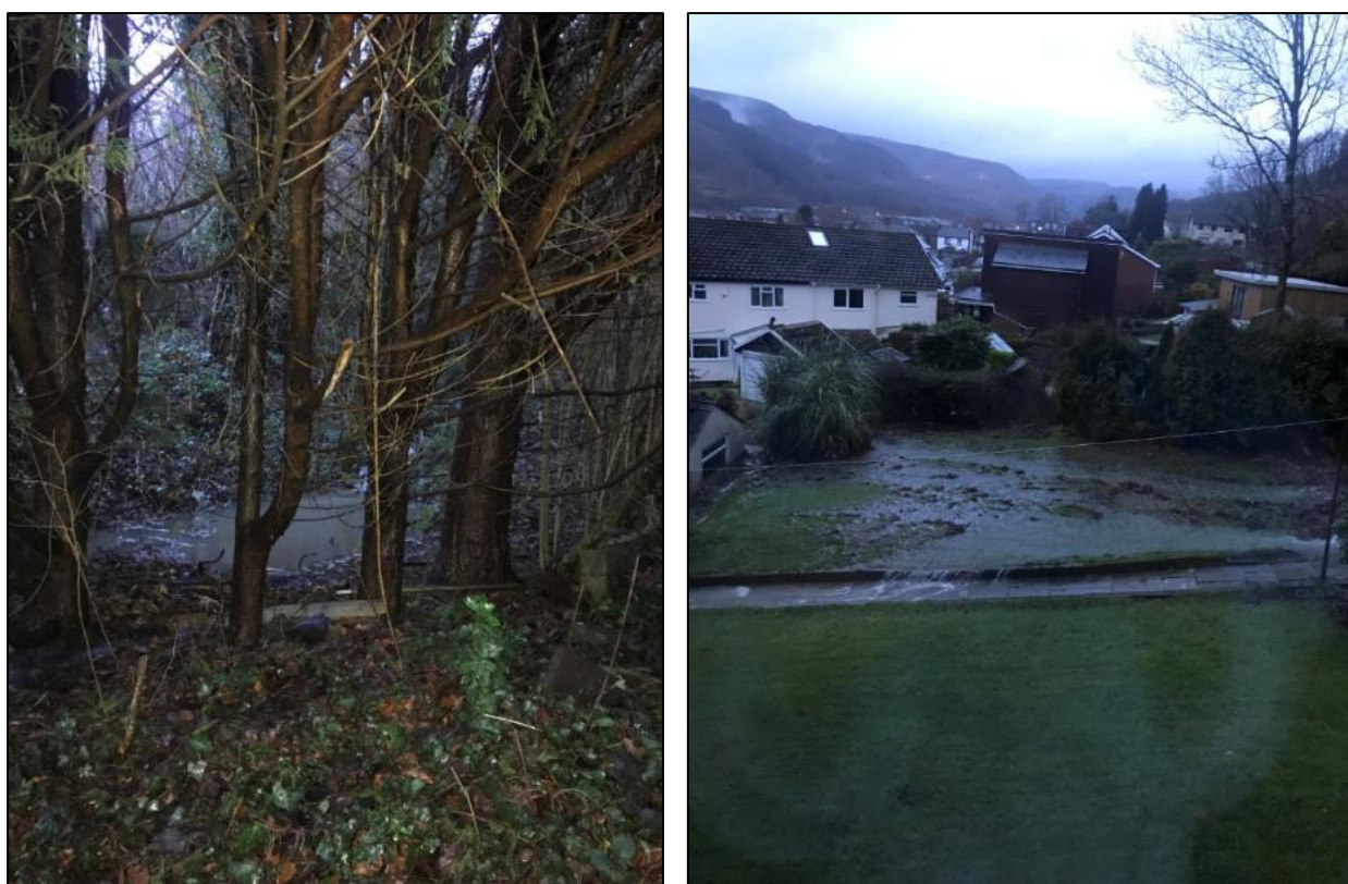
Figure 10: Evidence of 'Culvert Inlet 4' surcharging during Storm Dennis (left) and evidence of surcharging flows travelling through the garden of a private property towards the park space downstream (right) (images provided by resident)
